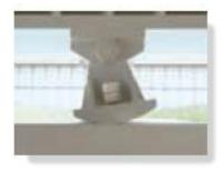
Roller supports are free to rotate and translate along the surface on which the roller rests. The surface can be horizontal, vertical or sloped at any angle.
