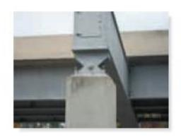
A pinned support can resist both vertical and horizontal forces but not a moment. They will allow the structural member to rotate, but not to translate in any direction.
